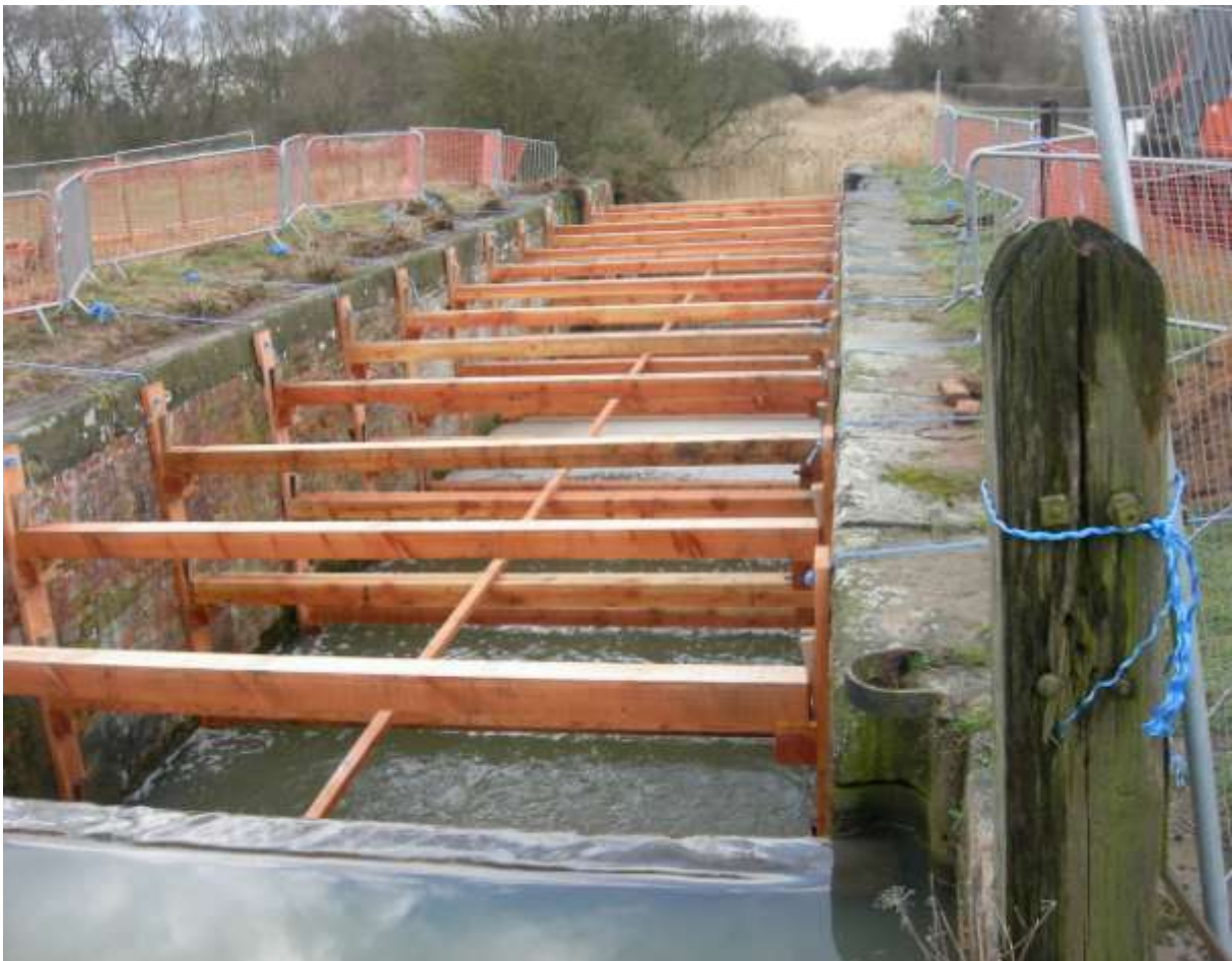
Sandhill Lock with bracing in place
