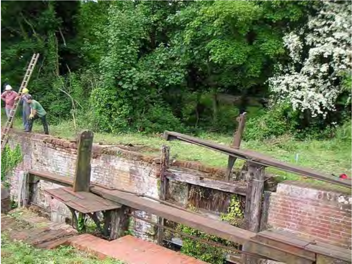
Briggate Lock. With iron balance beams
