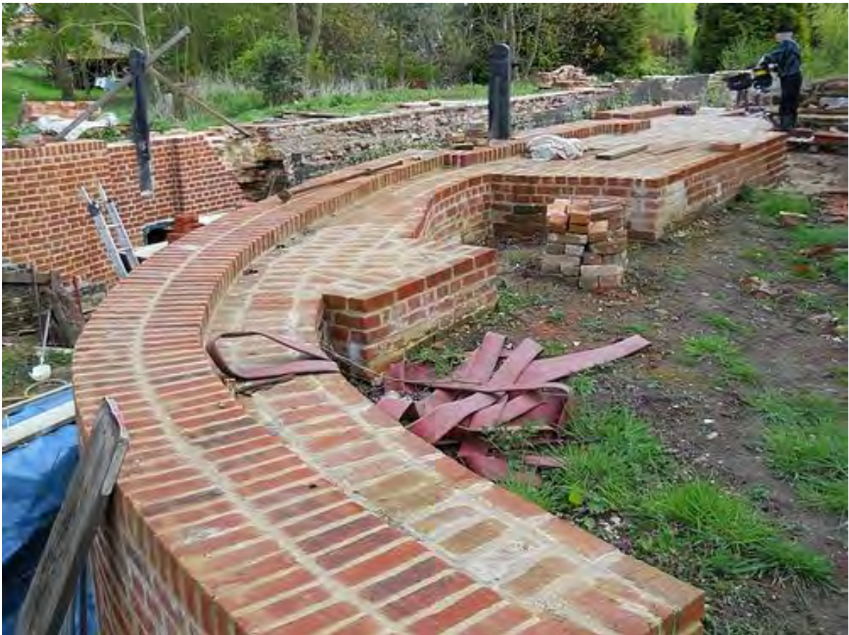
New brickwork on the Upper Canal at Bacton Wood
