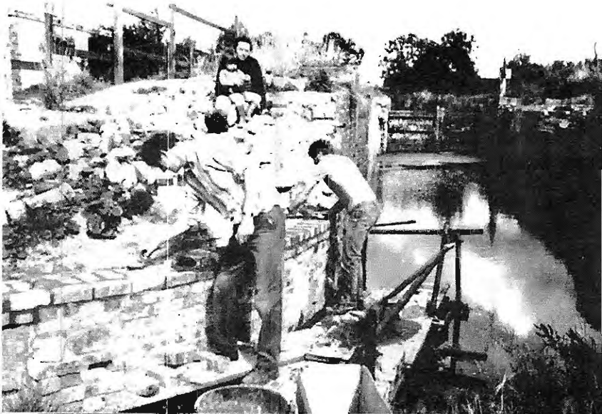
TOP LOCK - REBUILDING THE WING WALL
