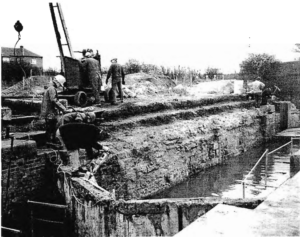
above: Coates Lock - offside wall and remains of cascade and old gates
