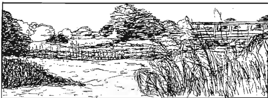
Melbourne Arm and the Bridge that Collapsed during 1983
